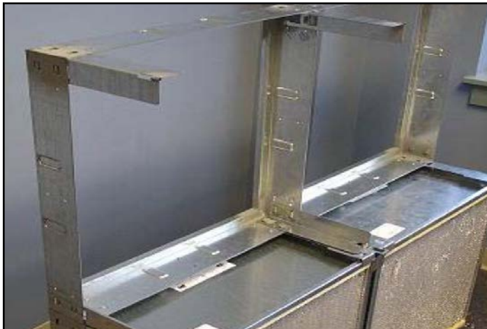
Figure 118: Frame with Leg Extensions Installed
