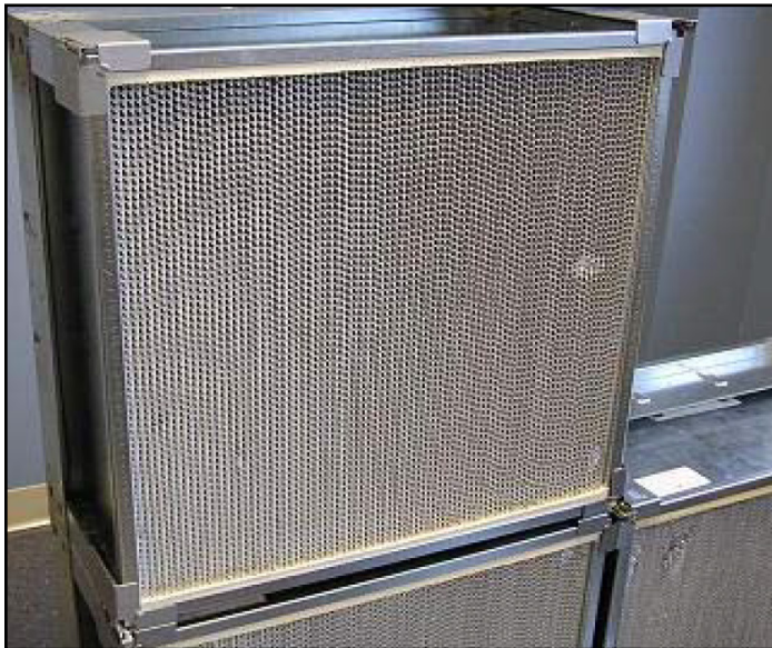
Figure 125: Properly Installed Filter Inside of the Frame
