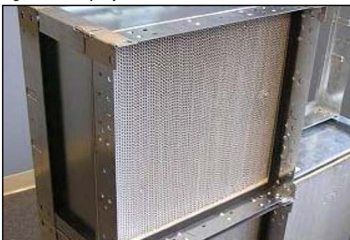
Figure 130: Properly Installed HEPA Filter
